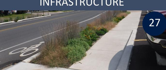
Green Stormwater Infrastructure (GSI) in sidewalks, medians, and curb extensions collects stormwater runoff and filters it through special soil and plants before it soaks into the ground or is released slowly back into the sewer system.
