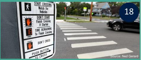
A pedestrian countdown signal includes an accessible push button, appropriate signage, and a pedestrian signal that indicates remaining walk time. Fixed, rather than actuated, signals are most preferred in urban areas.
