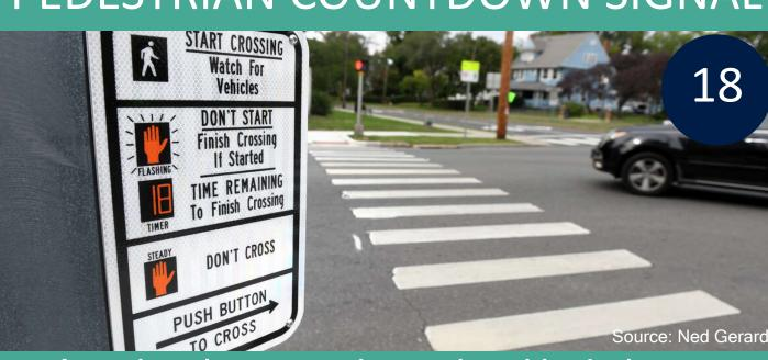
A pedestrian countdown signal includes an accessible push button, appropriate signage, and a pedestrian signal that indicates remaining walk time. Fixed, rather than actuated, signals are most preferred in urban areas.
