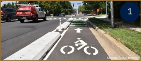
A separated bike lane is within the street rightof-way and separated from motor vehicle traffic by a physical barrier, such as planters, flexible delineator posts, parked cars, landscape median, or a mountable curb.
