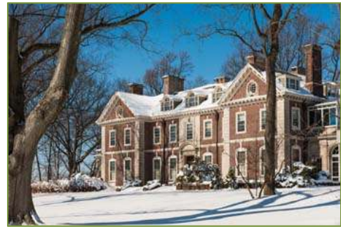
Figure 2-5: Ardrossan Estate in Radnor, PA
