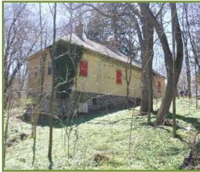
Figure 2-22: Side View Showing Roof Cupola
