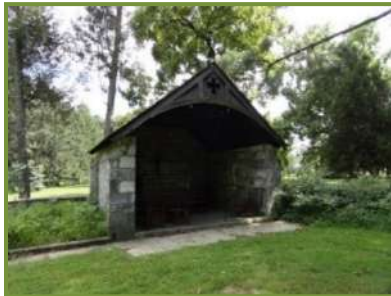
Figure 2-28: Side View of the Stone Grotto
