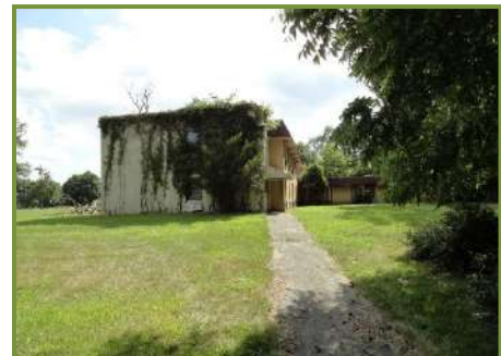
Figure 2-25: Side Wall of Convent Covered in Vines
