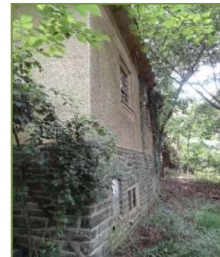
Figure 2-20: Foundation of ‘The Barn’
