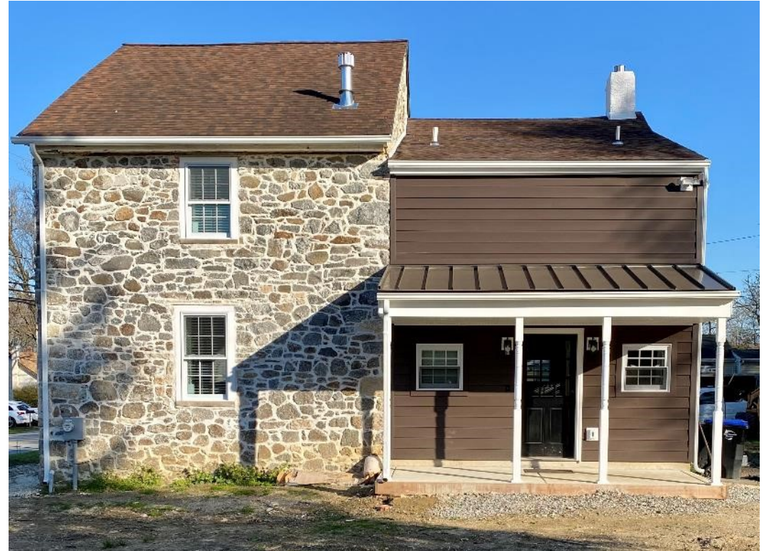
Siding on addition, new porch added
