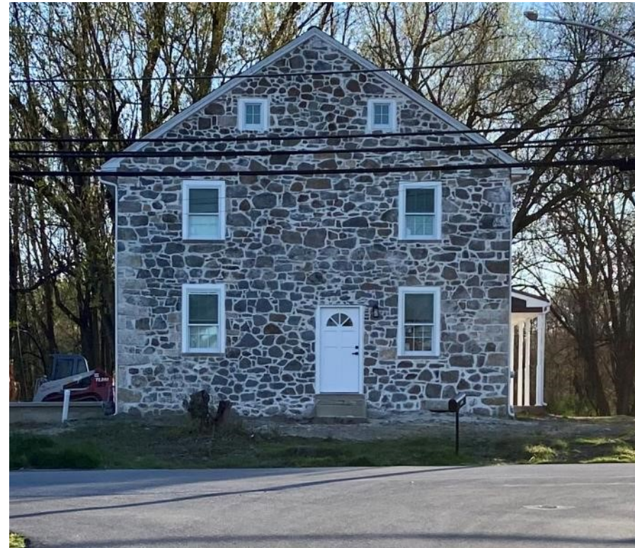
After stucco removal and stone repointing
