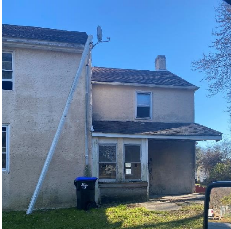
Rear addition with ca. 1960 porch
