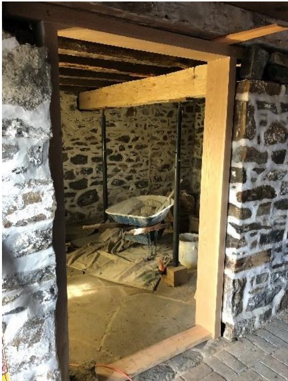
New Beam, Door Frame and Floor
