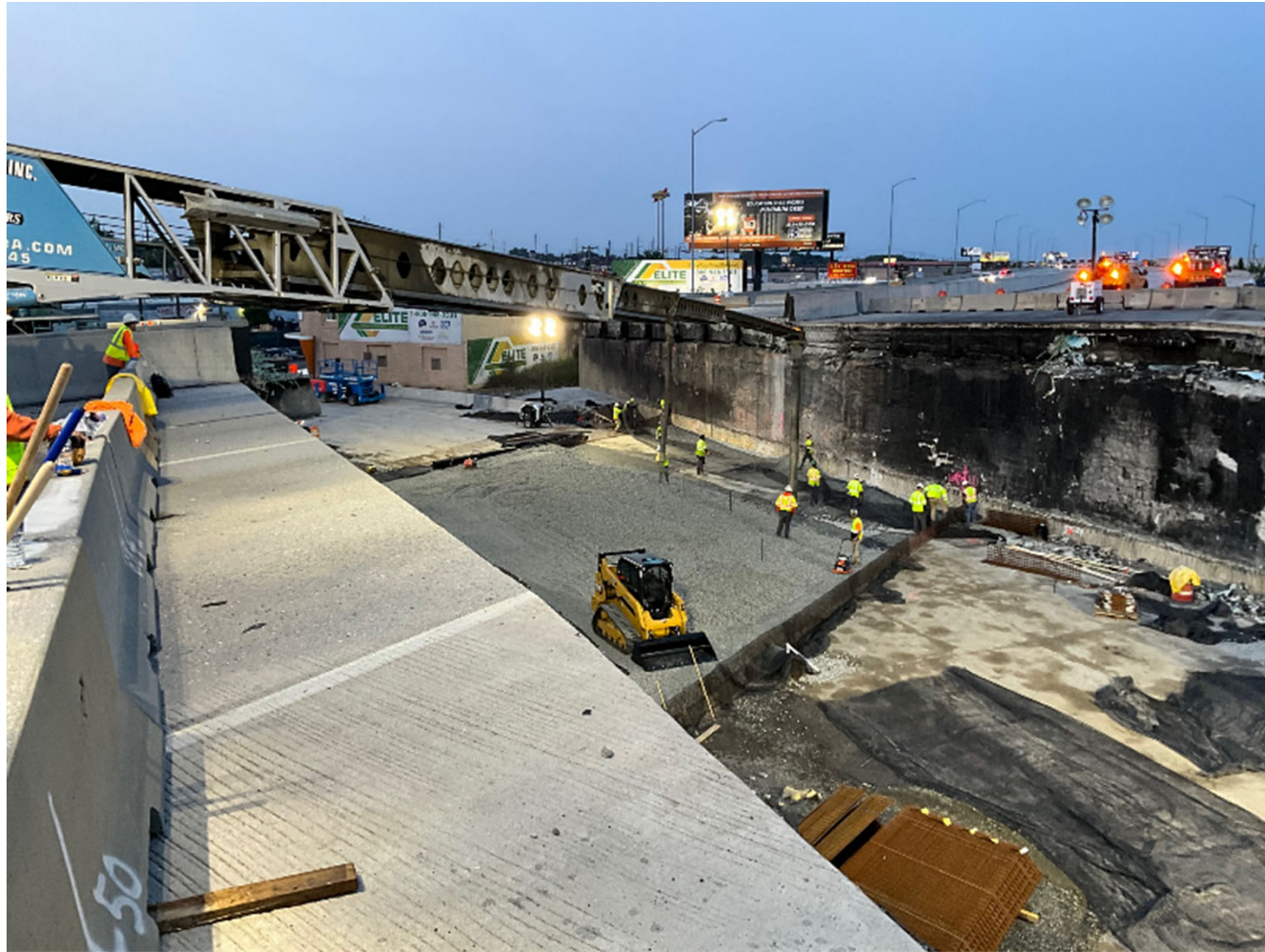
First lifts of MSE Wall
