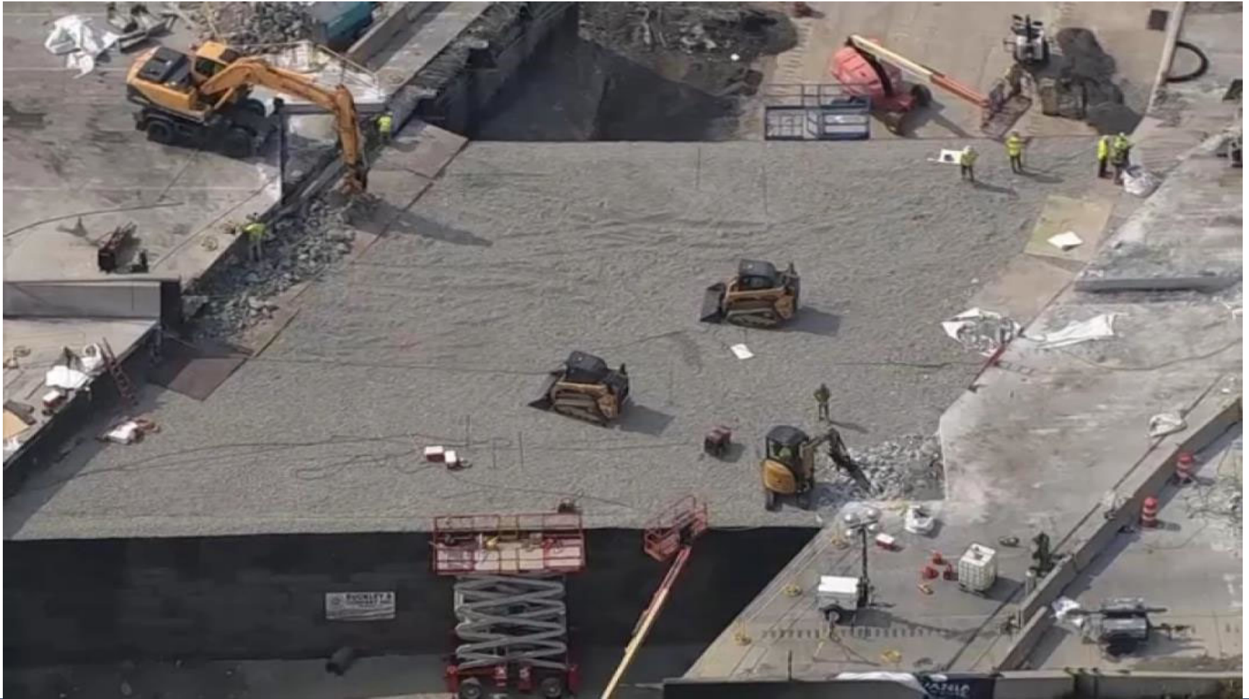
I-95 Prior to subbase and paving
