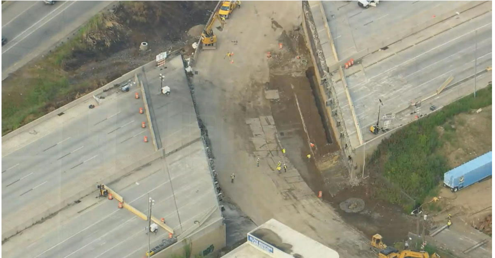
June 15 th 4 days after collapse
