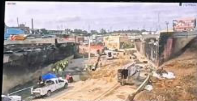
C_De_portable_1 N MLInor St on ramp
