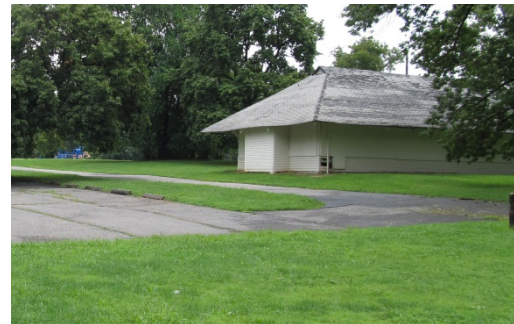
Figure 7-19: Pavilion / Maintenance Building
