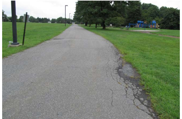
Figure 7-11: Access drive looking north
