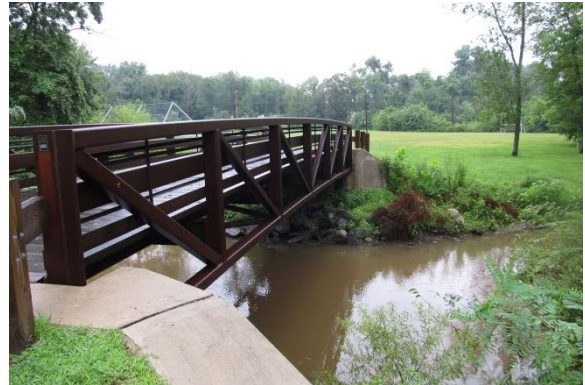
Figure 6-10: Six pedestrian bridges over Crum Creek
