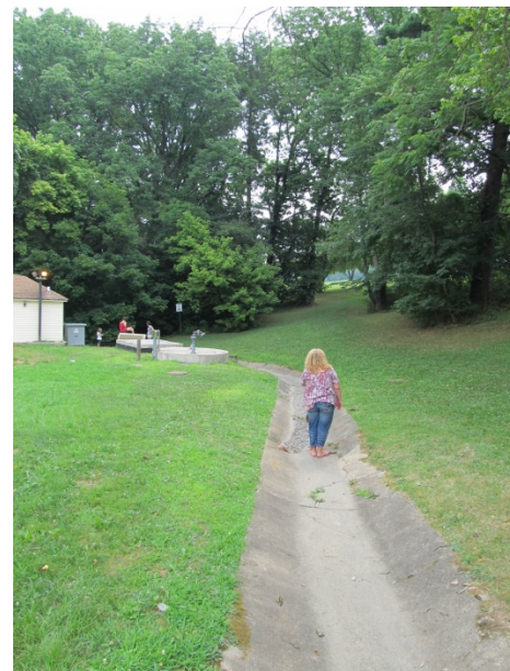
Figure 5-4: Concrete drainage channel
