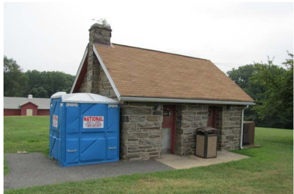
Figure 5-12: Restroom Facilities (b)
