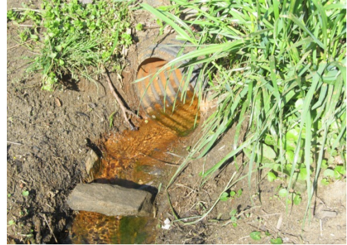
Figure 4-6: Stormwater outlet along Darby Creek
