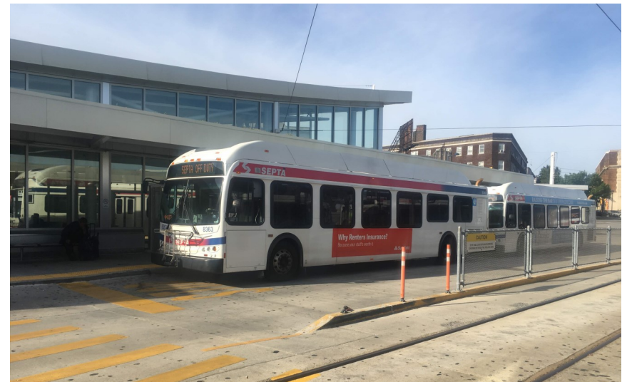
69th St station
