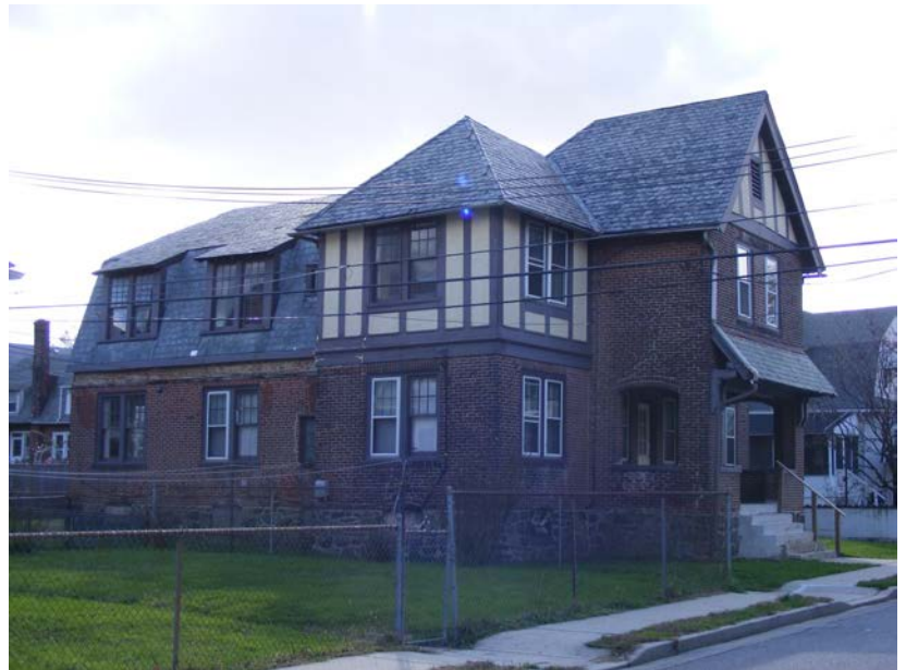
Note Original Slate Roof
