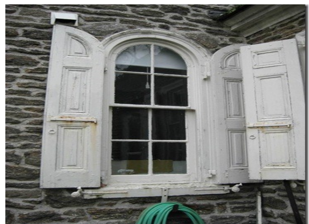
Wood shutters attached to round window opening
