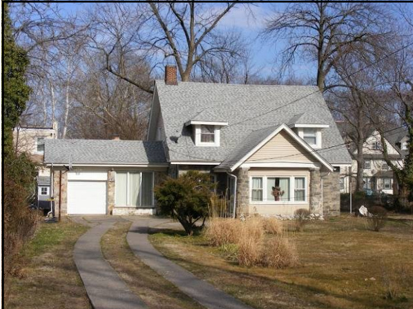
Using driveway strips increases ground cover
