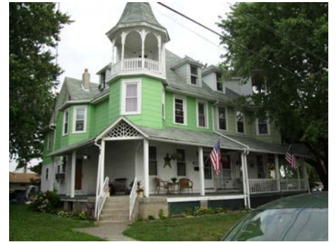
Hipped roof with cross-gable and turret
