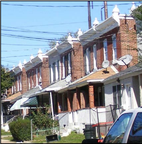
Roof cornices highlight these row of twins.
