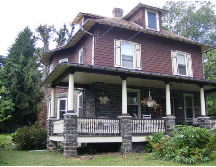
Full-width, one-story porch with stone supports
