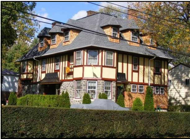
Wide eaves on roof line and multiple dormers
