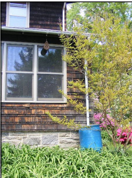
Downspout into rain barrel.
