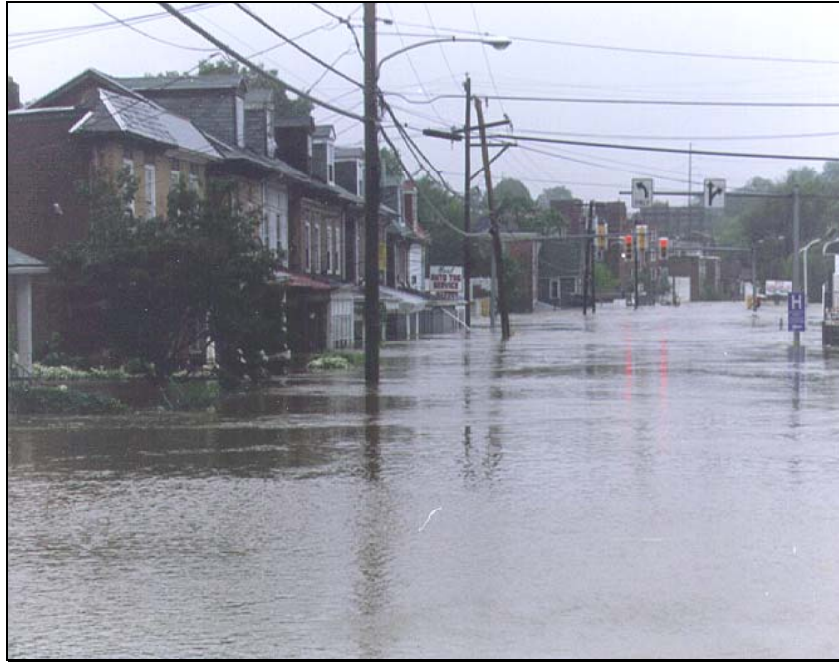
Figure III-11 Overbank Flooding – Darby Creek, Borough of Darby
