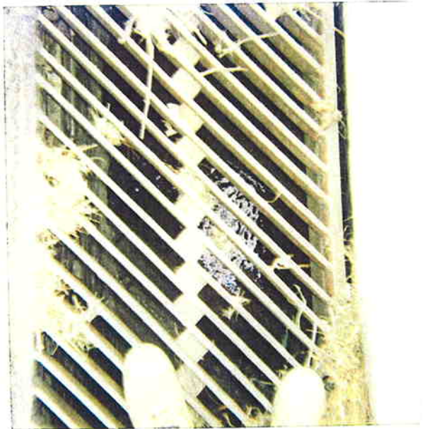
115 Meadow - Storm Drain Direct to Box Culvert - Beatty Run # B3
