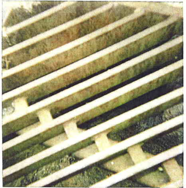
Taylor Drive - Storm Drain to Box Culvert, Beatty Run # B1
