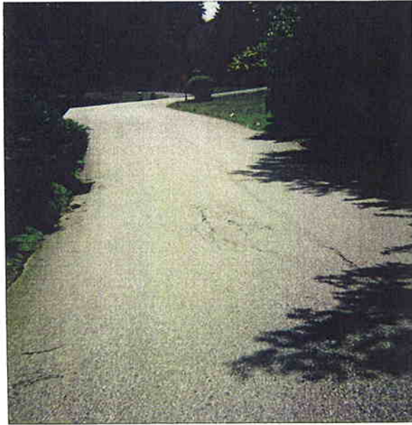
Bt 13 Devon At Waterford Direct to Box Culvert
