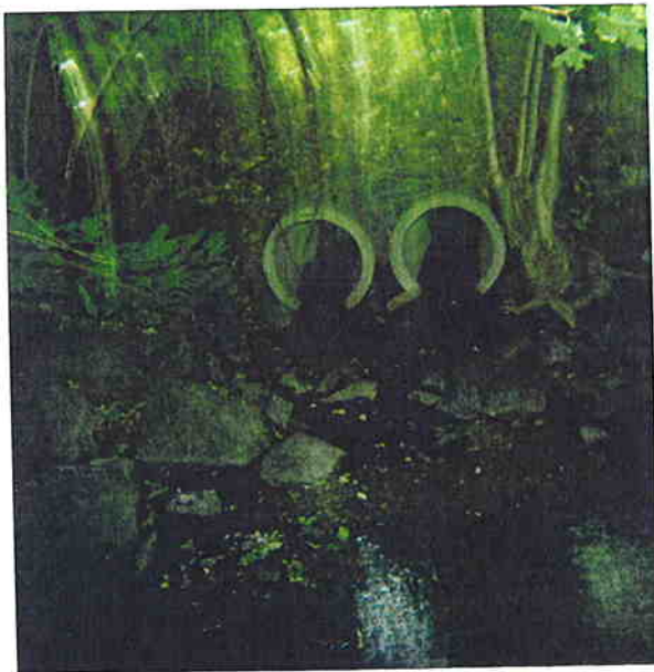
D17 - Avondale @ end of concrete sidewalk with Blue Route overhead to Dicks Run
