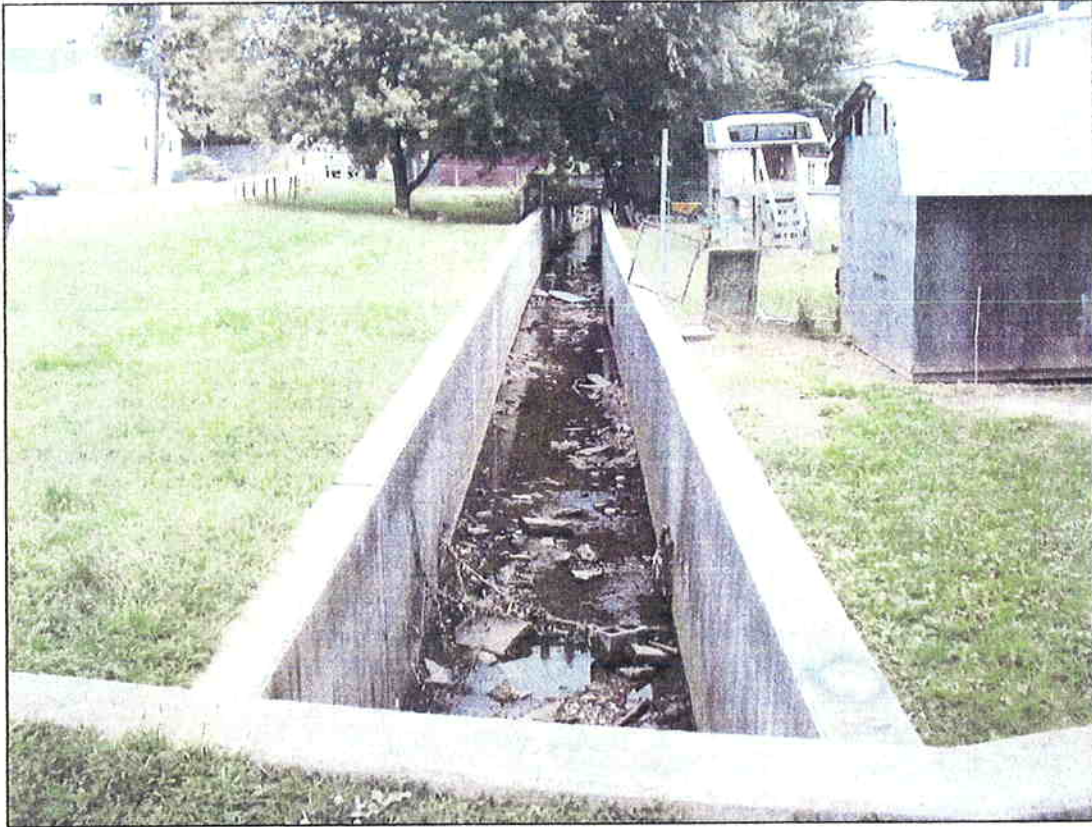
J-3, Walter St: concrete channel
