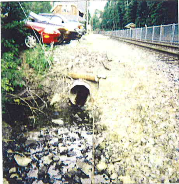
D7 - Possum Hollow to Dicks Run - Train Station
