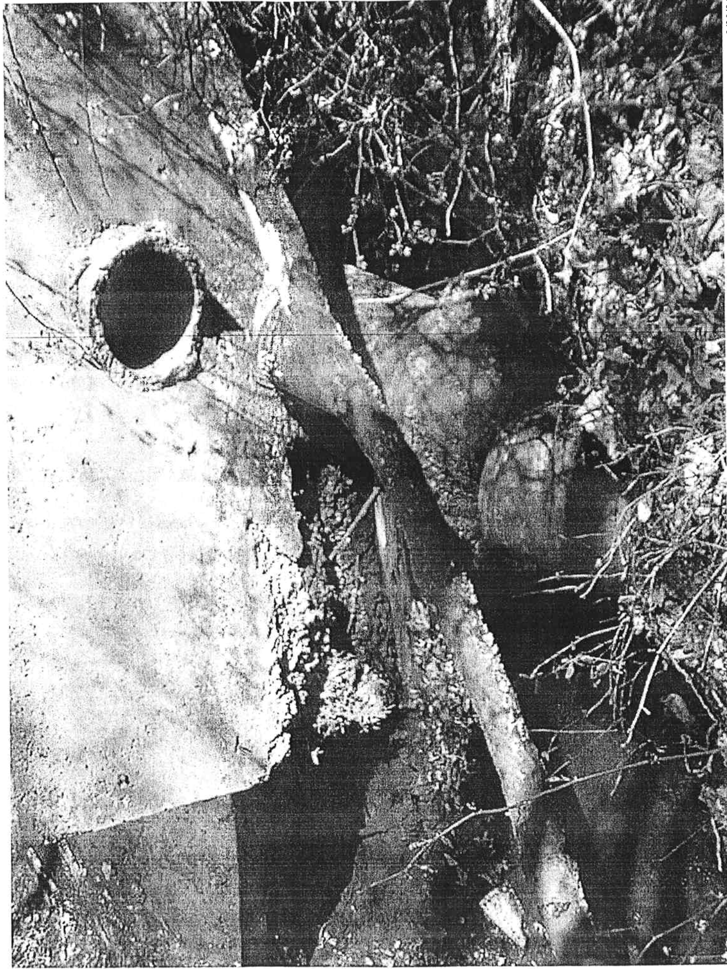
Pipe Swale #45 - Swarthmore, Little Crum Creek Disk #4 - Photo #9
