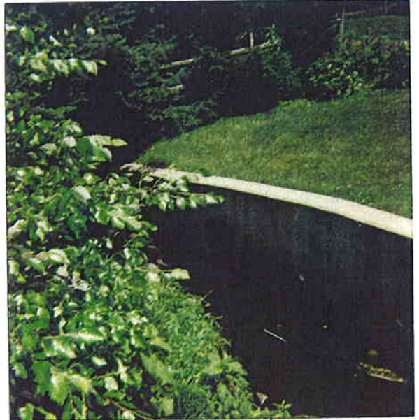
Plush Mill @ Dogwood d 2 exit pipes D 2
