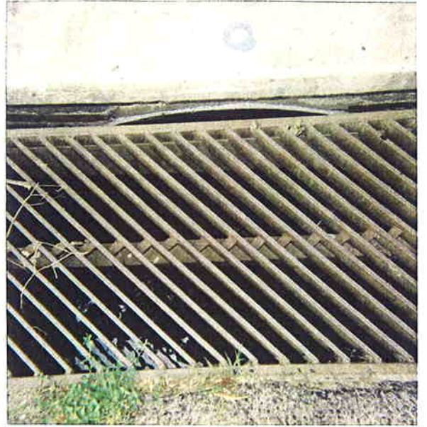
216 LAUREL LANE Direct to Box Culvert
