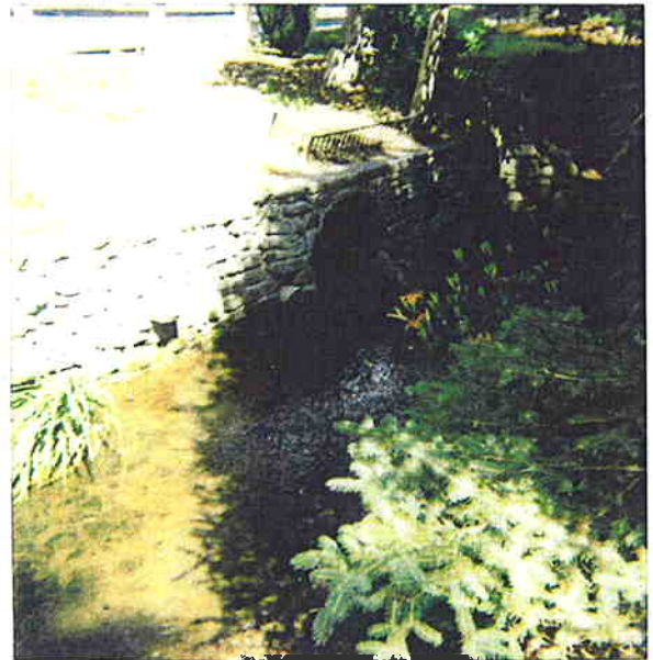
Avondale @ Kershaw to Dicks Run D 12
