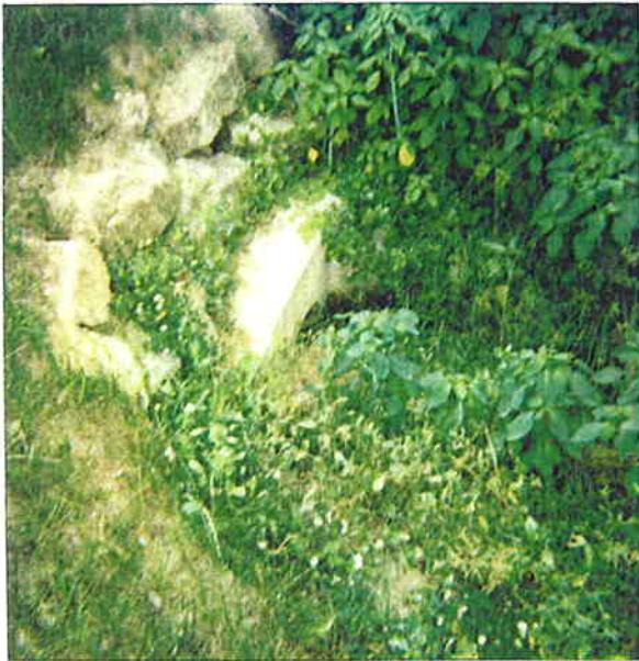
Dewey Lane - New Development 18" Pipe to Beatty # B2
