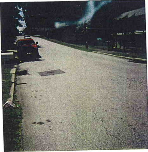
BT 10 532 Georgetown TO Box Culvert
