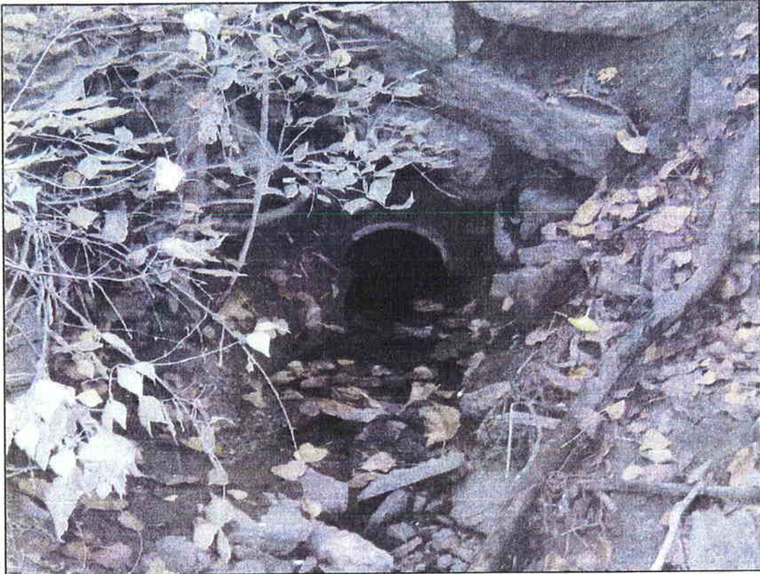
J-2, Chester Pike: outfall pipe feeding orange channel
