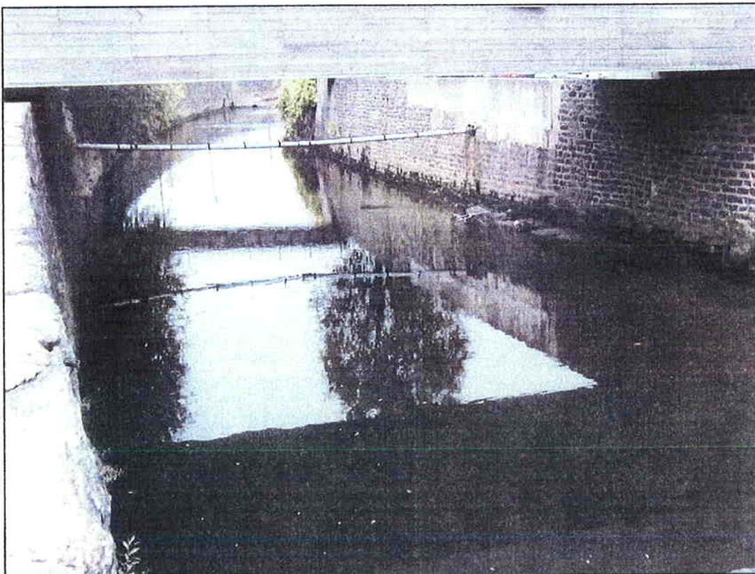
J-1, Baldwin Towers: lined channel
