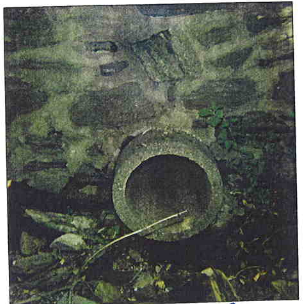
From Knoll to Dicks Run D 4 - 18" concrete
