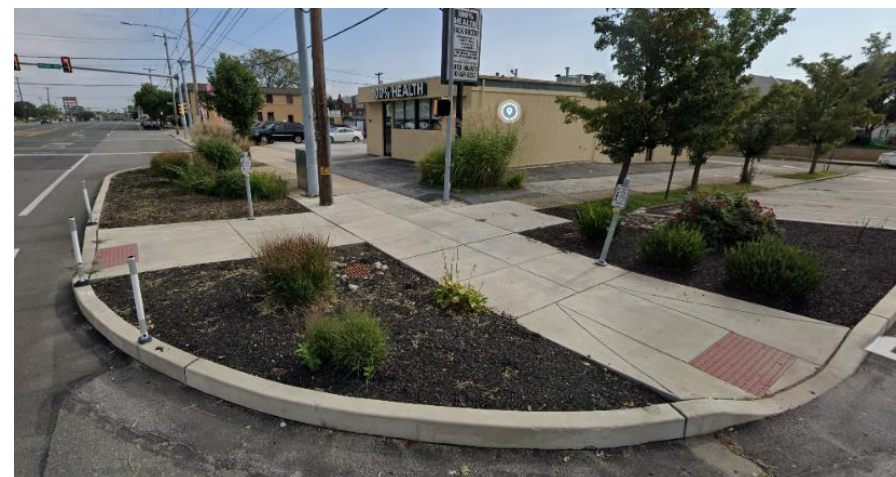
Figure 6-4: Bumpouts at Brainerd Blvd, across from the Sharon Hill Trolley Station
