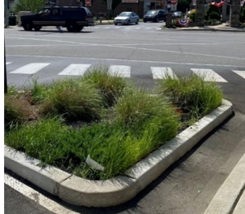
Figure 3-7: Bump Out and Gateway Feature on Winoa Ave, Norwood
