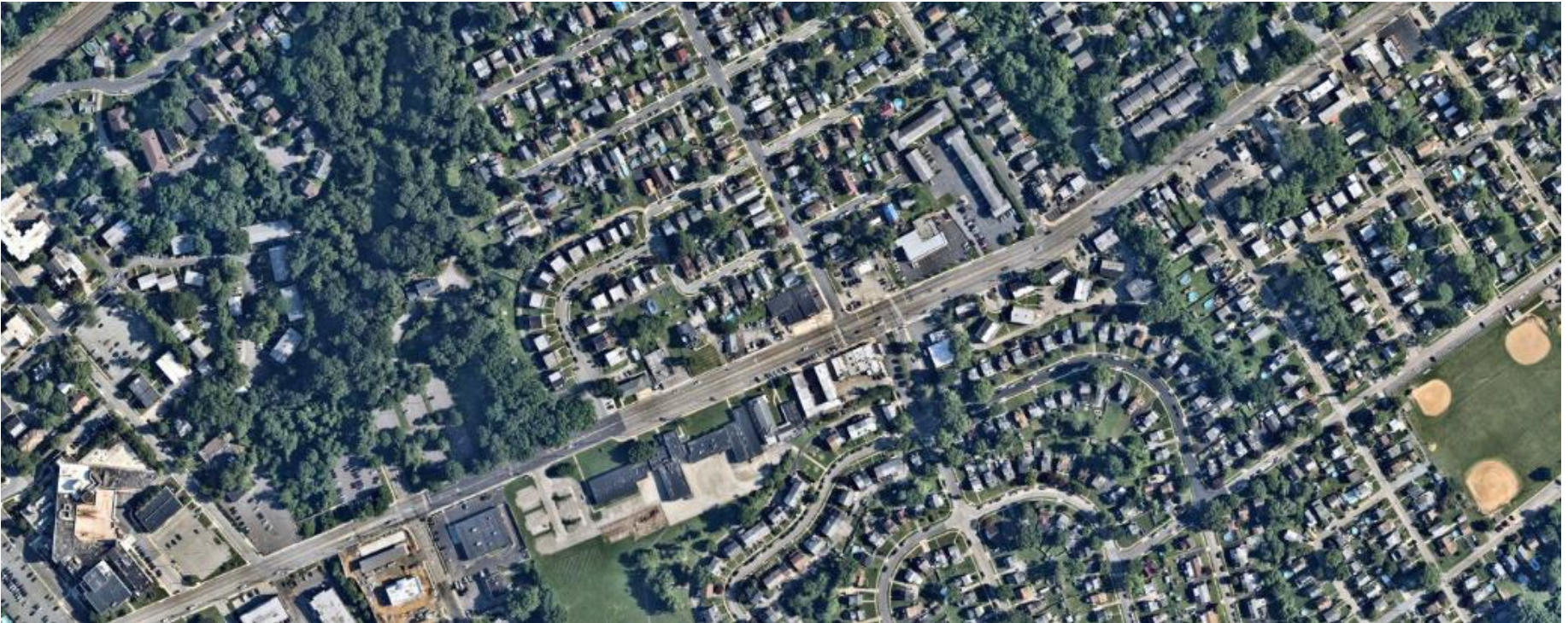
Figure 2-1: Aerial view of Chester Pike (Ridley Park & Prospect Park)
