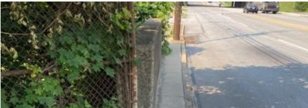
Figure 6-2: Narrow sidewalk segment crossing Little Crum Creek.
