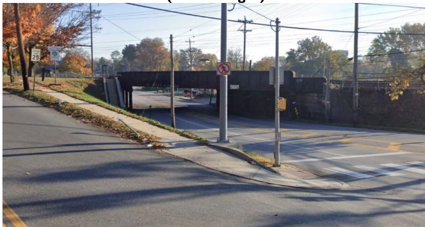
Figure 3-2: Ridley Avenue (Left) and Chester Pike (Center/Right)
