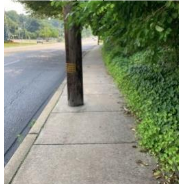
Figure 6-1: Utility pole blocking sidewalk across from Taylor Hospital
